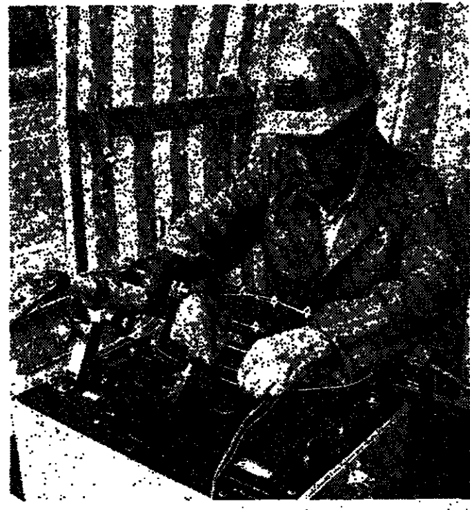
Installing the new generation of telephone lines requires skills closer to microsurgery than to traditional cable laying. In the picture above, British Telecom technician John Crick is joining two pieces of fibre optic cable beside the AS in Bedfordshire. Telecom is laying the latest "monomode" fibre between Luton and Milton Keynes. A pair of these glass strands, each thinner than a hair, carries up to 2,000 phone calls.
